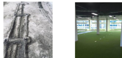
6. Kazakhstan factory flooring
